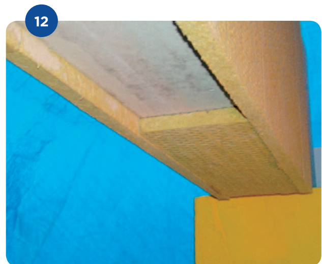
The flange is glued in the end
