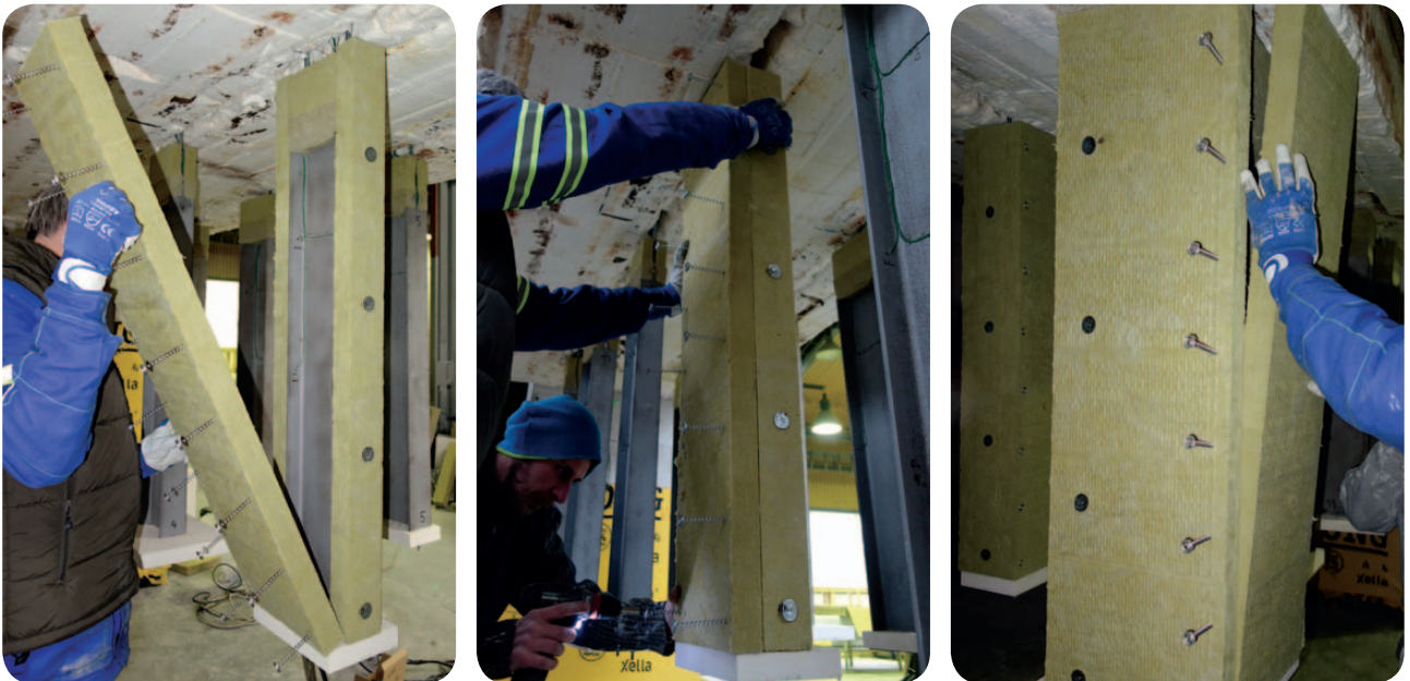
Fig. 6 Both methods can be also combined – important is to keep the distances (between pins 300 mm and between Fire Screws 150 mm)
