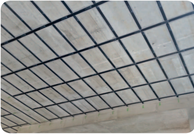
Fig. 17 Carbon fiber reinforced lamellas before fire protection
