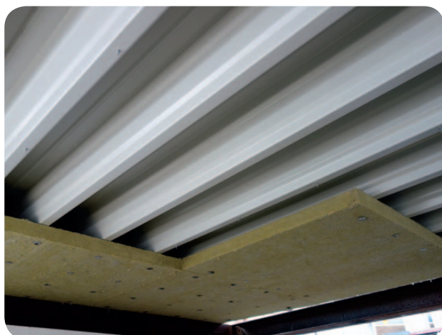
Fig. 10 System Isover FireProtect® for fire protection of corrugated steel is characterized by light weight and small height, but also a direct fixing to the corrugated steel without need of help of suspension construction
