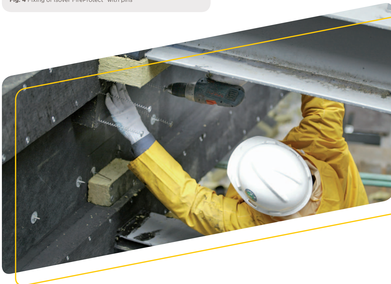
Fig. 4 Fixing of Isover FireProtect® with pins
