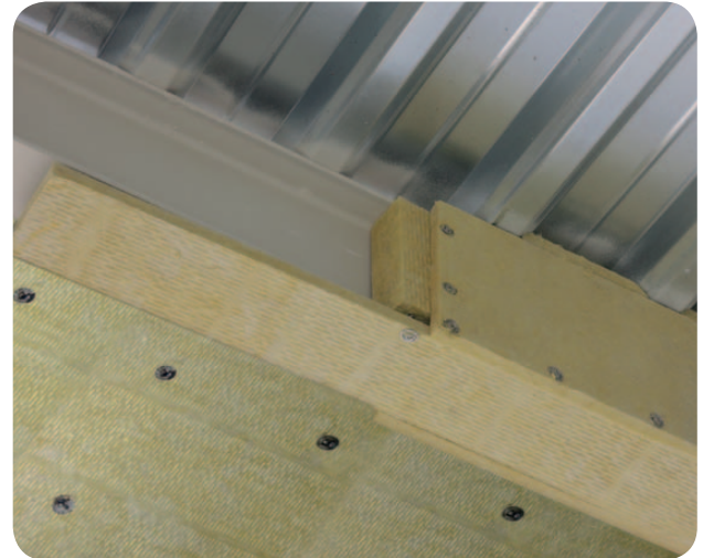
Fig. 15 The four side fire protection of a steel beam (using the Isover FireProtect® 150 slabs to backfill a trapezoidal profile)
