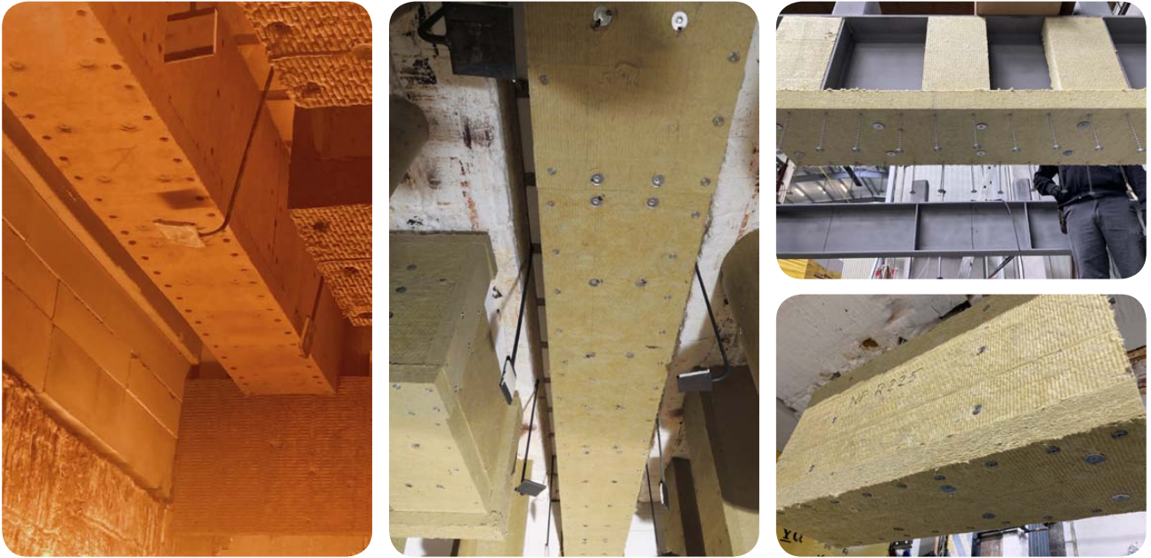
Fig. 5 Bottom slab with insulation thickness \geq 50 mm is fixed to the lower flange of the beam both with Fire Screws and welding pins.
